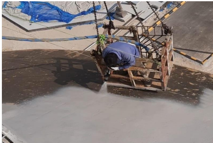
Our reference in Alkhuber (KSA): Azizia sewage treatment plant
