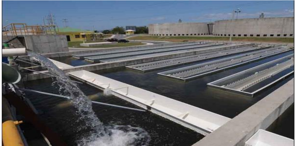
Our reference in Alkhuber (KSA): Azizia sewage treatment plant
